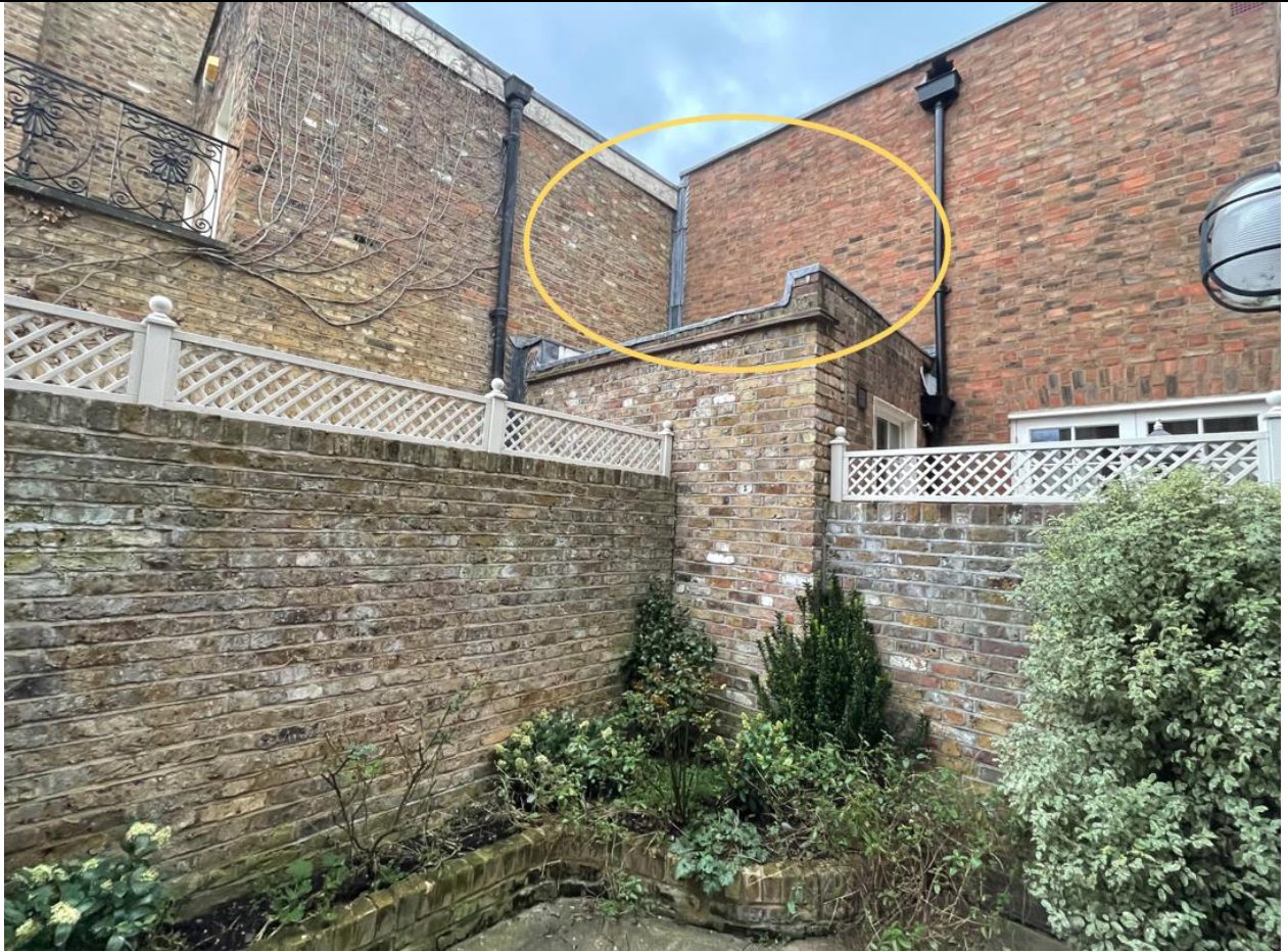
Approximate position of proposed extension highlighted (viewed from neighbouring garden).
